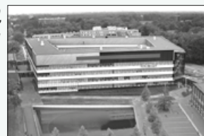
● 2010 Multi-purpose building 'Carre' J. Hoogstad
