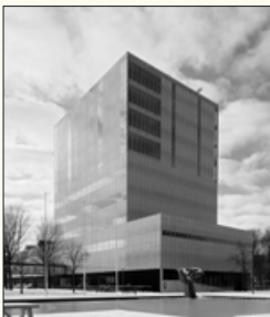
● 2002 Redevelopment 'T-Hoog' into Faculty of Architecture 'Vertigo' DiedererDirix
